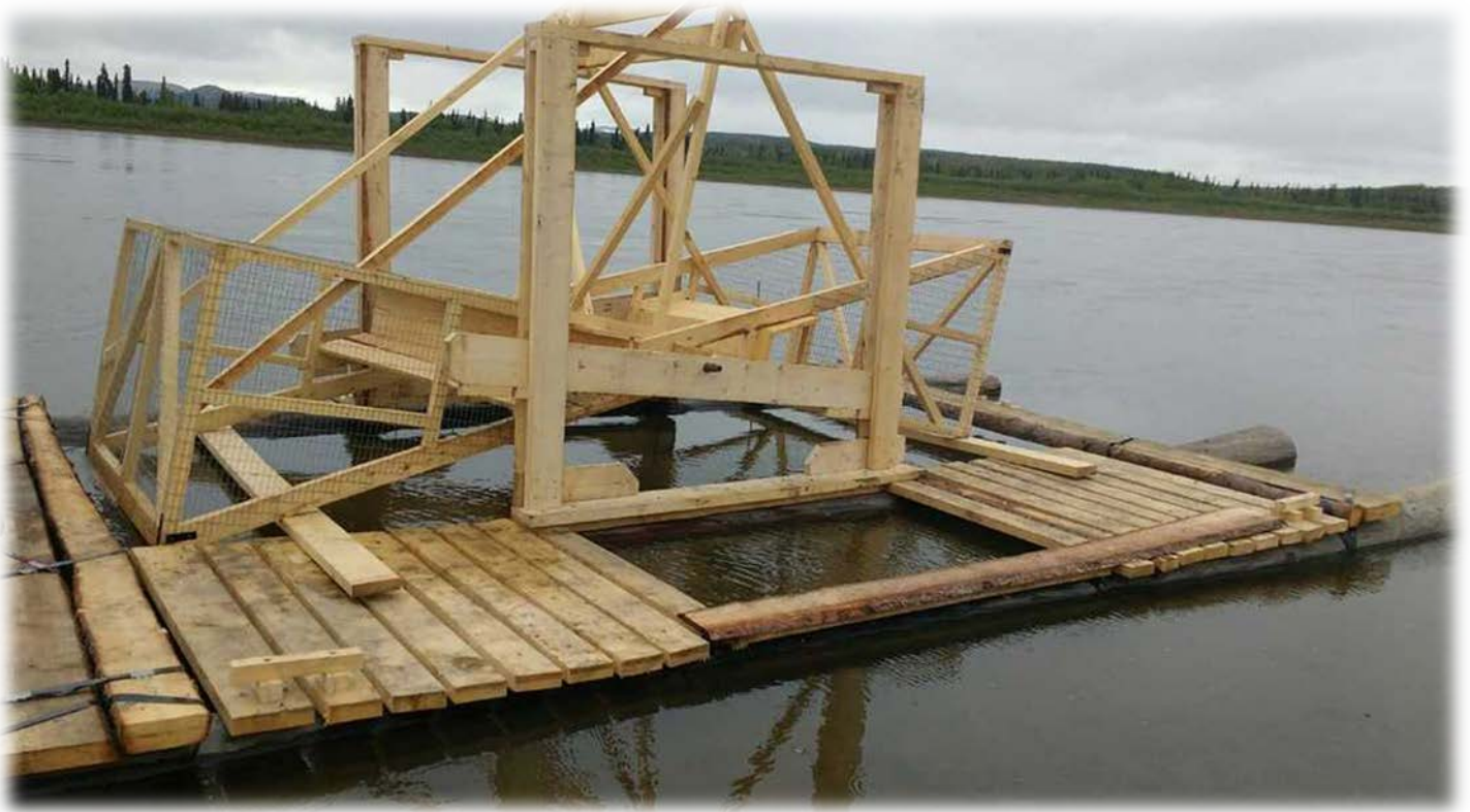
Then the ladders, live boxes, and baskets are installed
